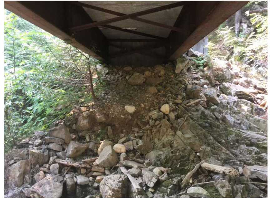
Right Bank Abutment when facing downstream
