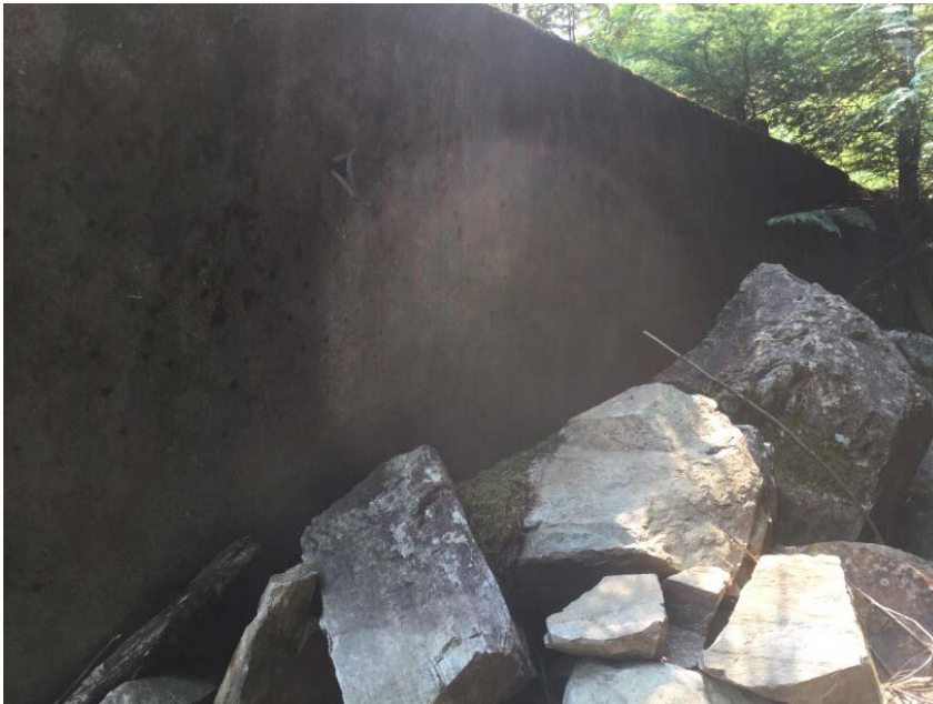
Upstream right approach wingwall
