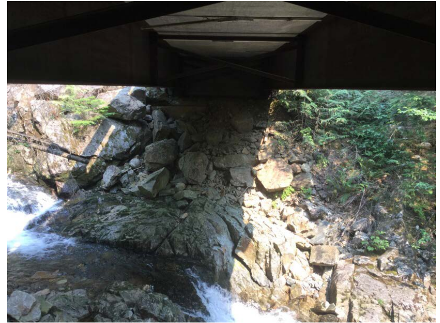
Left Bank Abutment when facing downstream
