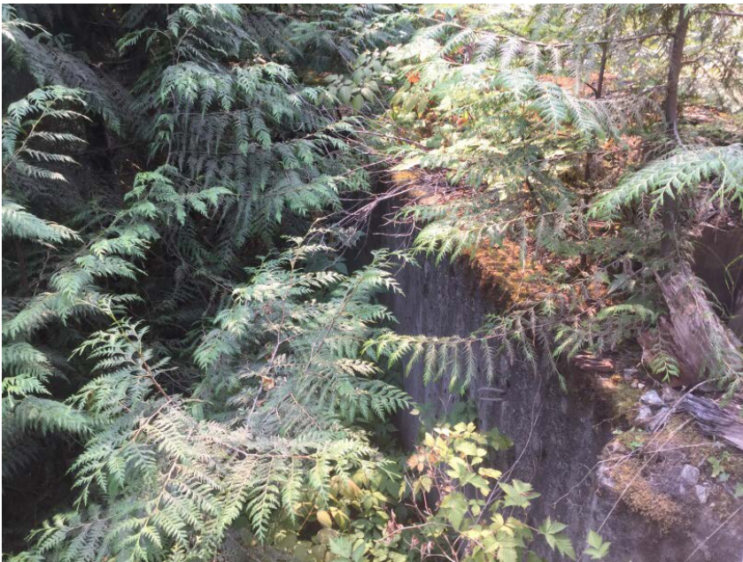
Downstream right bank wingwall
